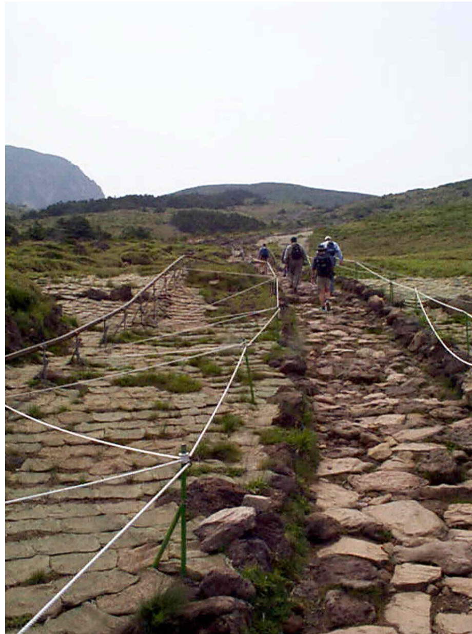
Large paving stones and hessian-like bags used for soil stabilisation, Orimok track
