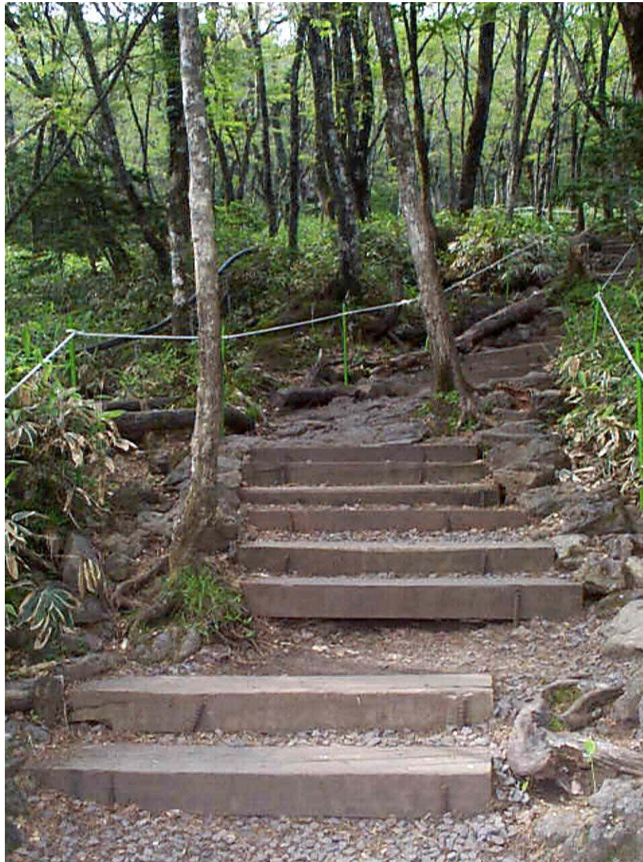
Hardwood steps and gravel used for soil stabilisation. Orimok track
