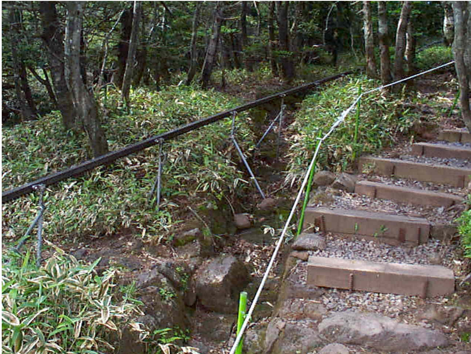
Monorail line, on left of picture, used for transport of rehabilitation materials. Orimok track
